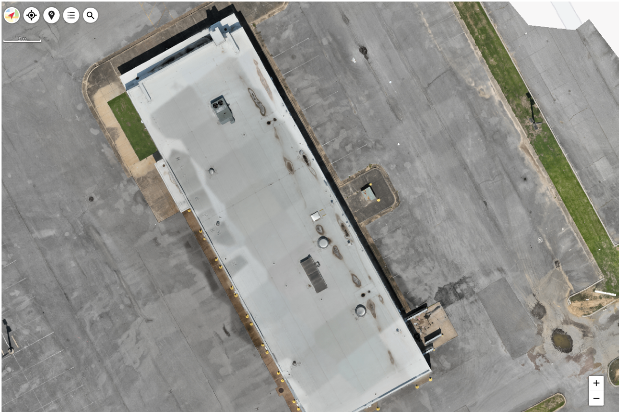
FIGURE 2: Close-range roof orthomosaic — Memphis-Area Commercial Property | July 2026
